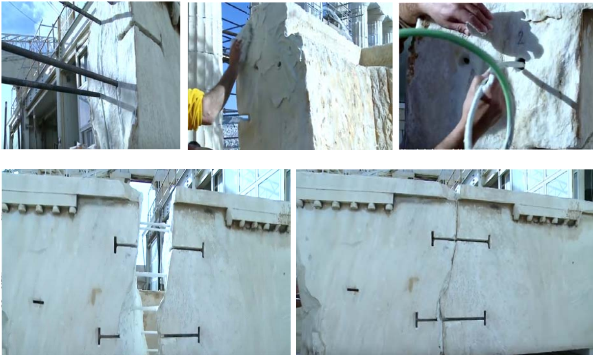
Figure 1: The main steps for the restoration of a marble epistyle [2].
